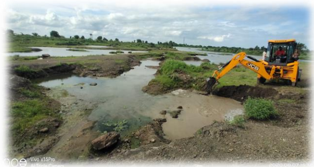
Stream desilting work in Lonje village
